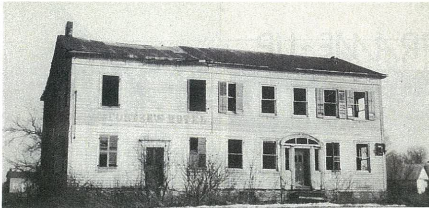
On its original site, 'Porter's Hotel' seemed a lost cause by 1965. Even so it was still an impressive building, worthy of recycling. Despite neglect, the original building (right) had weathered the years far better than the later addition (note serious sag in roof).
