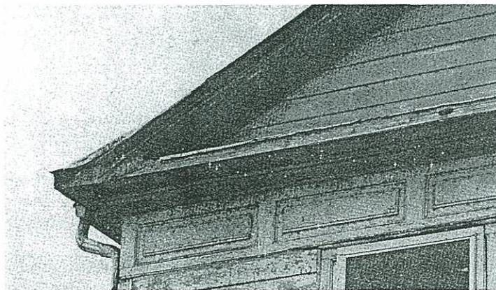
Whittier/Hall House, Consecon: a slightly different approach to the Greek Revival with mutules, and guttae represented by drilled holes, to the soffit.
